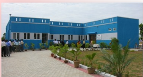
(Factory set up for dental composite production at Thiruporur at Kancheepuram District near Chennai )
